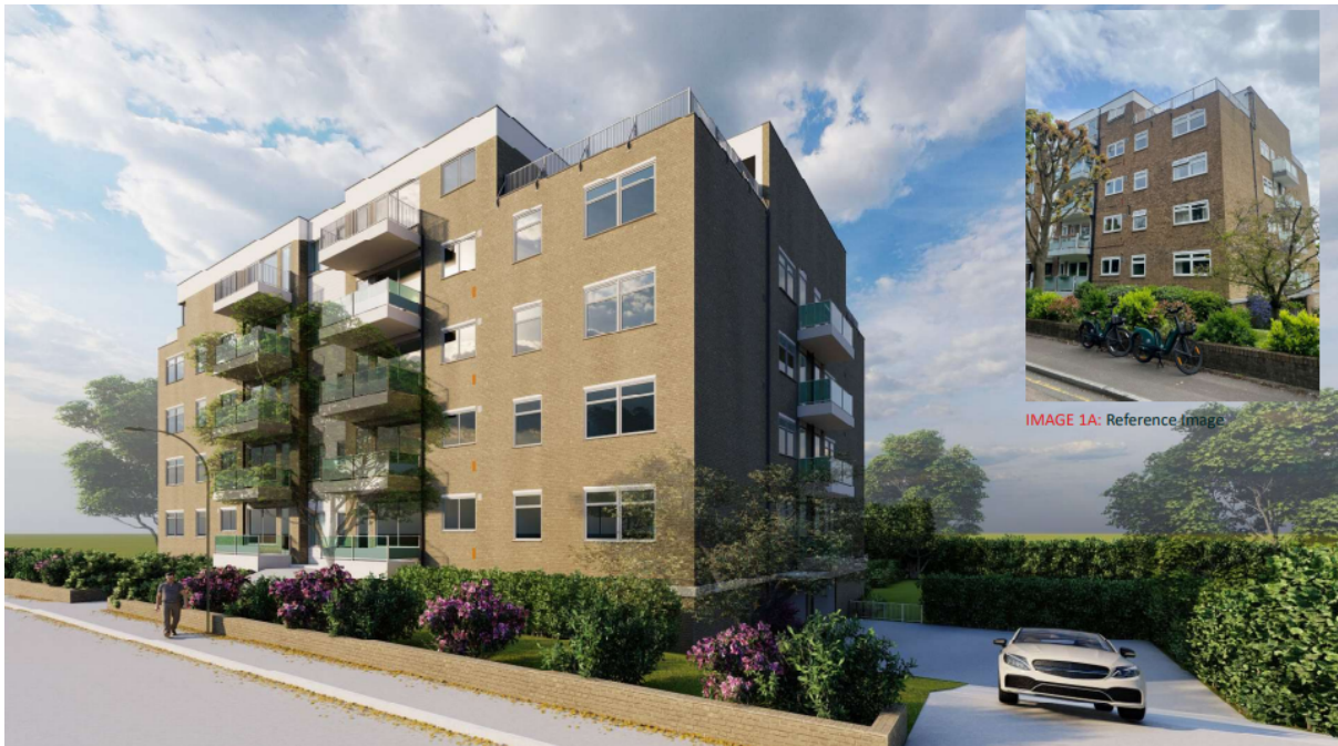
Fig 1 – the existing building with subject flat in foreground.
